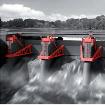
Hydro-electric power stations
